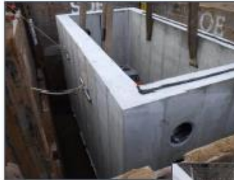
Vault Installation
